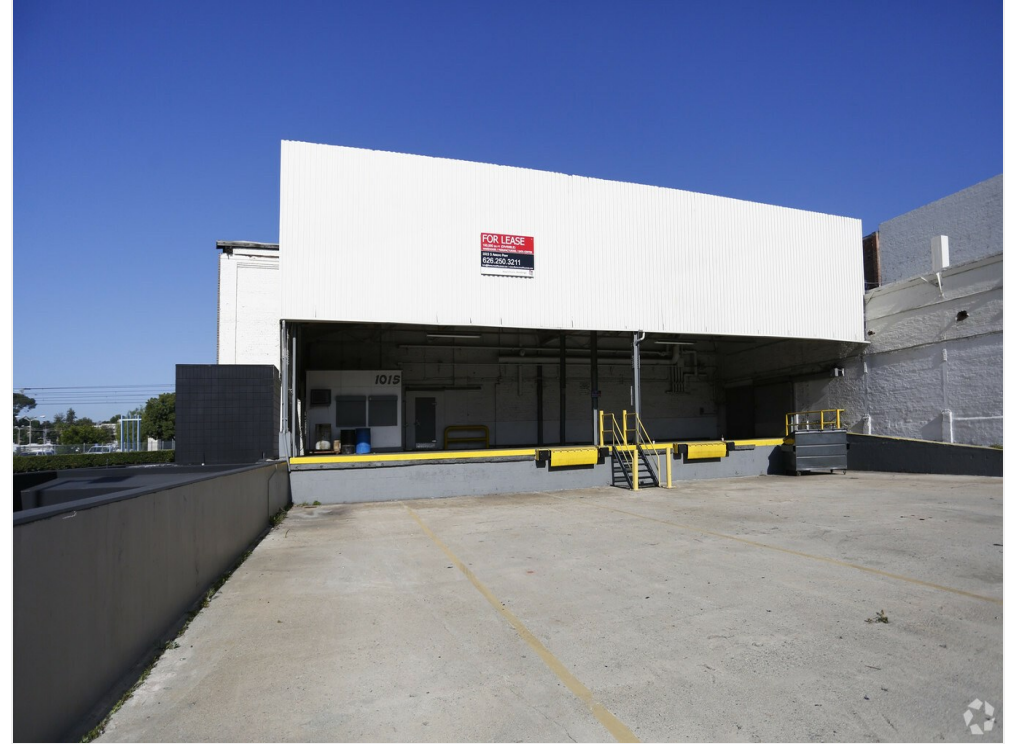
Main Loading Dock
